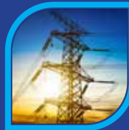
Enabling infrastructure (energy and digital)
